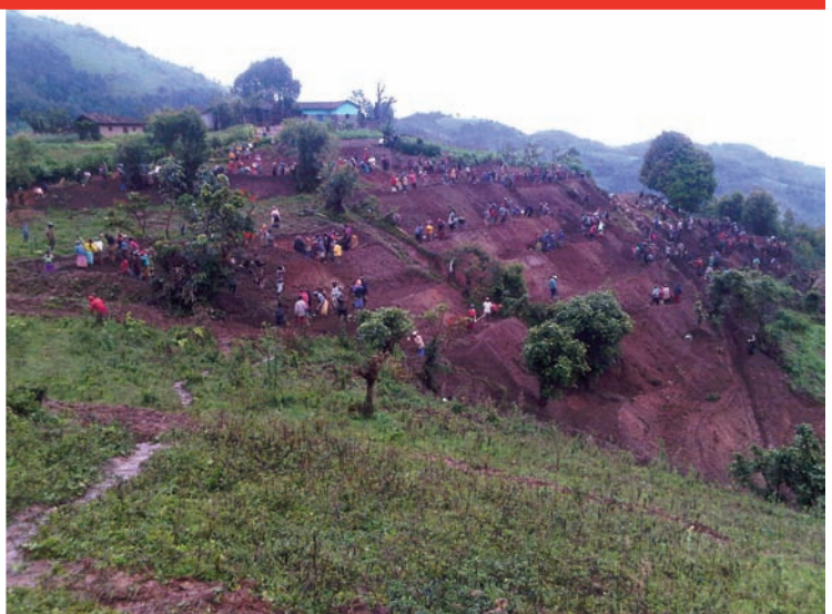
Worksite where farmers are constructing terraces.
